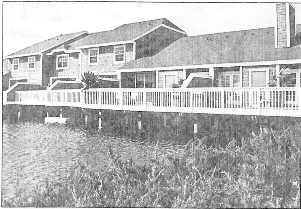
The charming model center is adjacent to the sparkling lake that serves as the community's focal point. All lakeside homes at Villas of Ocean Dunes have patios that extend out on wood pilings over the lake. Select Malayan coconut palms will accent the planned landscaping and will reflect gracefully in the water.
